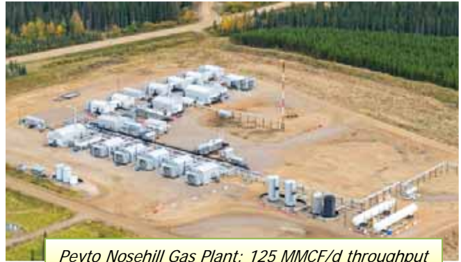
Peyto Nosehill Gas Plant: 125 MMCF/d throughput
