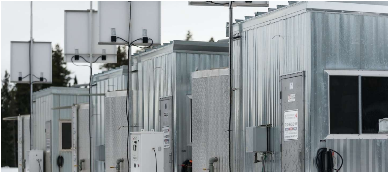
Typical Peyto multi-well pad measurement buildings equipped with solar panels, integrated water tanks, remote monitoring, and emergency shutdown equipment designed to minimize footprint while providing safe, reliable operations
