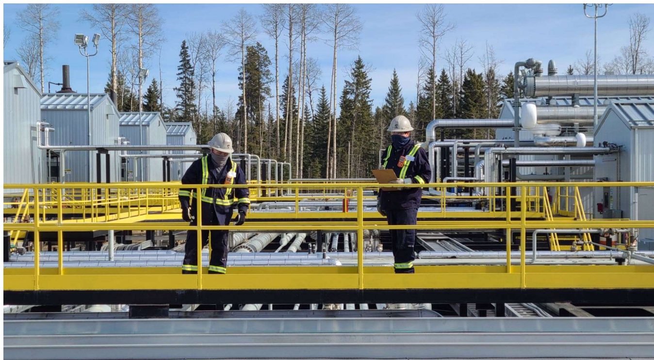
Operators at the Swanson Gas Plant conducting an inspection
