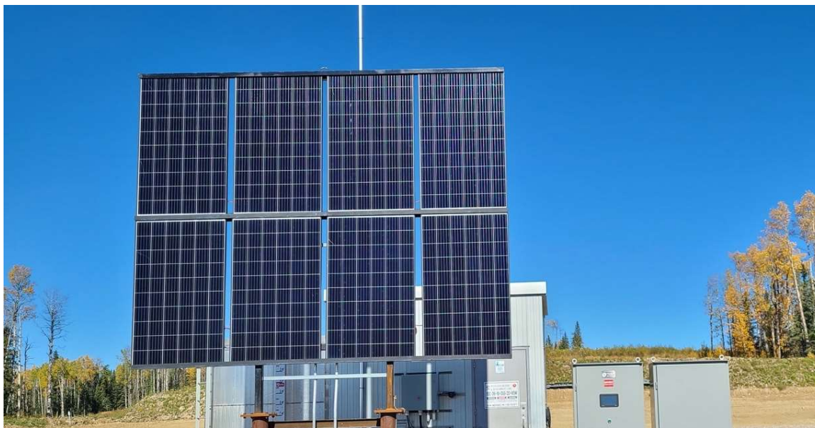
Peyto uses solar panels combined with battery storage to power electrical instrumentation and pumps to reduce Methane emissions
